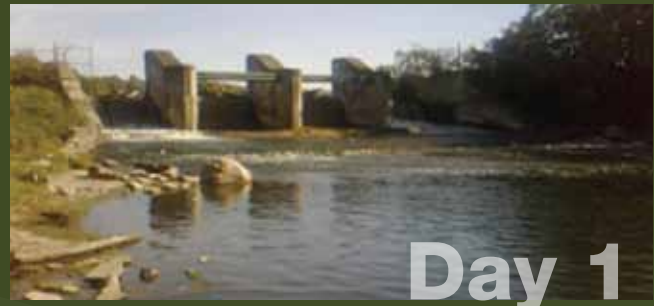
Series of photos taken during 2012 Shiawassee Town Dam drawdown.
