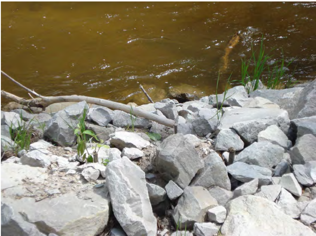
Live stakes placed in between the riprap for more stable root base
