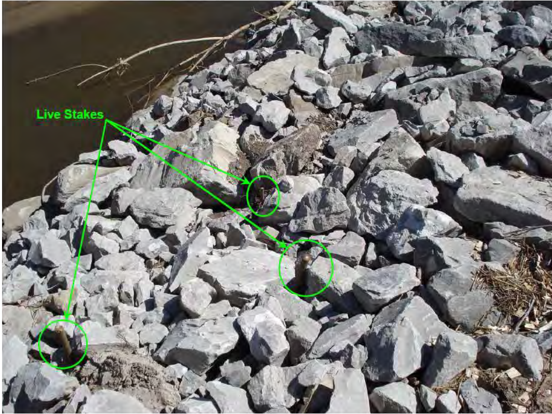
Live stakes placed in between the riprap for more stable root base
