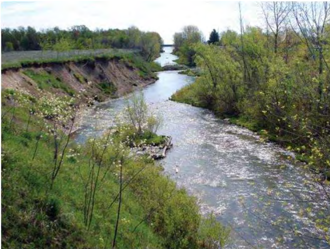
Figure 2: Pre-Project Conditions Example of severe bank erosion, log jams, and sediment bars in the downstream portion of the Whitney Drain.
