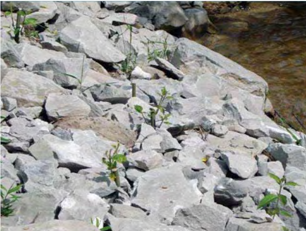
Figure 5: Live Stakes Live stakes taken from within the project area to create a root base to help stabilize the rock riprap bank.
