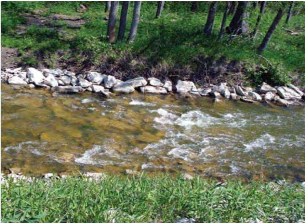
Figure 3: Typical Rock Riffle within the Whitney Intercounty Drain Example Rock riffle structure installed to stabilize the drain bottom by concentrating flow in the center of the channel.
