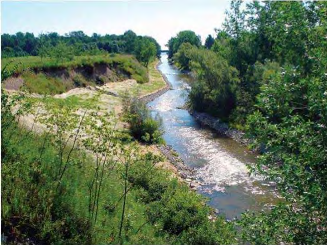
Figure 4: Channel Reconstruction Example of armoring banks with rock and floodplain benches to prevent future erosion and naturalize the area.
